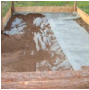
Used a weed barrier 2 feet below the site.
