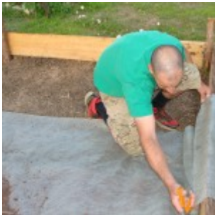
Trimming weed barrier.
