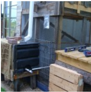
Davin created this rainbarrel to collect rain from the Greenhouse coop which runs into the 4 drip feeders inside the coop.
