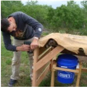
Davin stapling the burlap down to the frame
