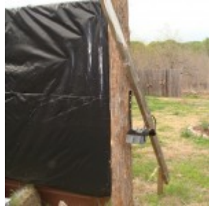
Securing the frame during cementing process.
