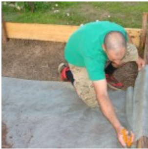
Trimming weed barrier.
