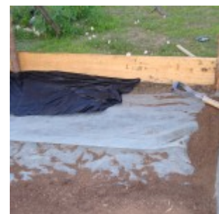
After digging the site we installed the frame.
