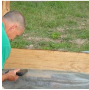
Staple gunned the weed barrier we purchased at Habitat for Humanity, Austin.
