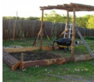
Half the bed is dug, frame is outlines, pergola constructed.
