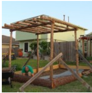
Support Beams used to secure Pergola Garden Bed into place.
