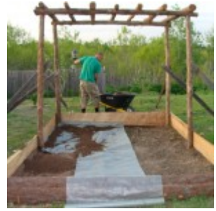
Laying dirt in bed.
